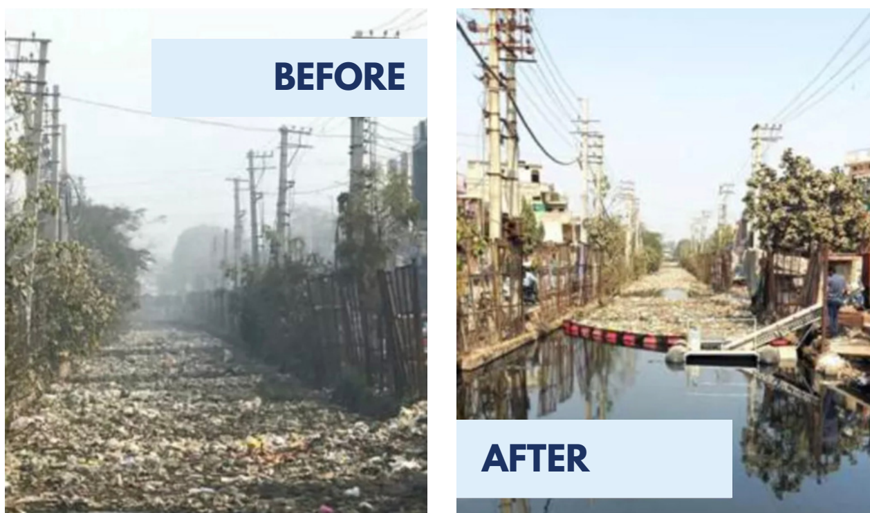
Figure 7. Comparison of debris retention effect with a River Boom installed in a canal in Hyderabad, India.*
