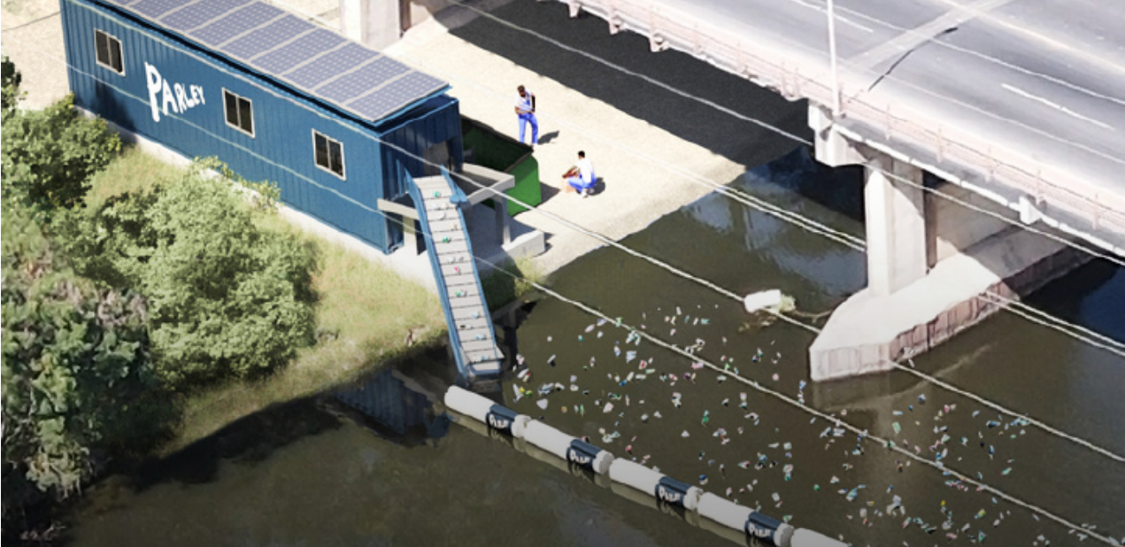
Figure 5. River Boom installed in the Ozama River, Dominican Republic.
