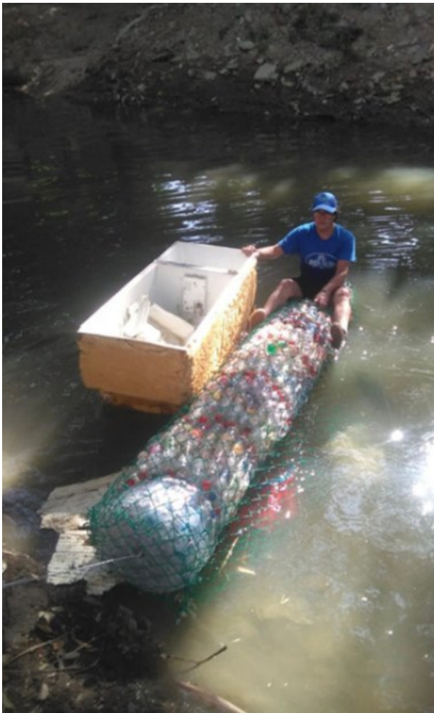
Figure 21. Biobarrier installation in Rio, Santa Marta.
